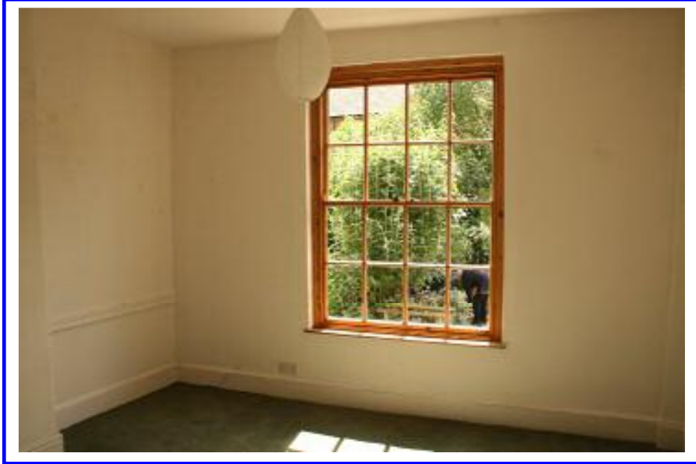
A Typical Office (Ground Floor Rear)
