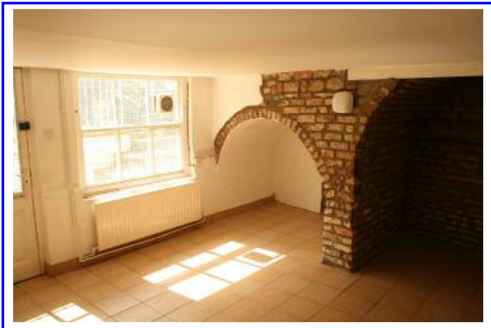
Basement (Rear Office)
