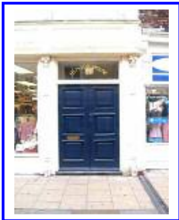
Main Entrance Door
